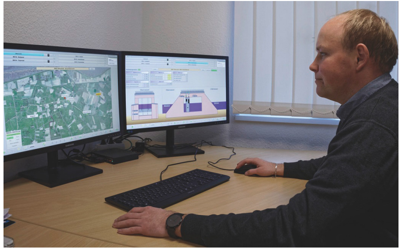
Everything under control: thanks to the automation and telecontrol technology, association technician Helge Schreiber can monitor and control the connected tidal sluice gates from the control center in Garding.
