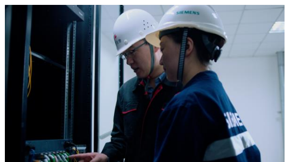
Digital solutions from Siemens ensure a safe and stable production environment for Jinyu Bio.
