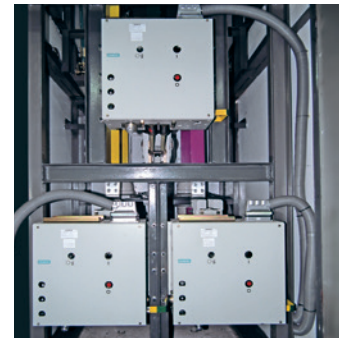
Example of a retrofit installation of the 3AH37 90 kA circuit-breaker
