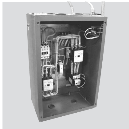
Fig. 3 Automatic Star Delta Starter (ASD)
