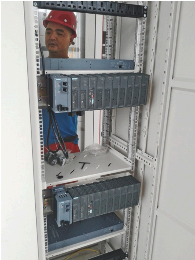
Two SCALANCE switches during installation
