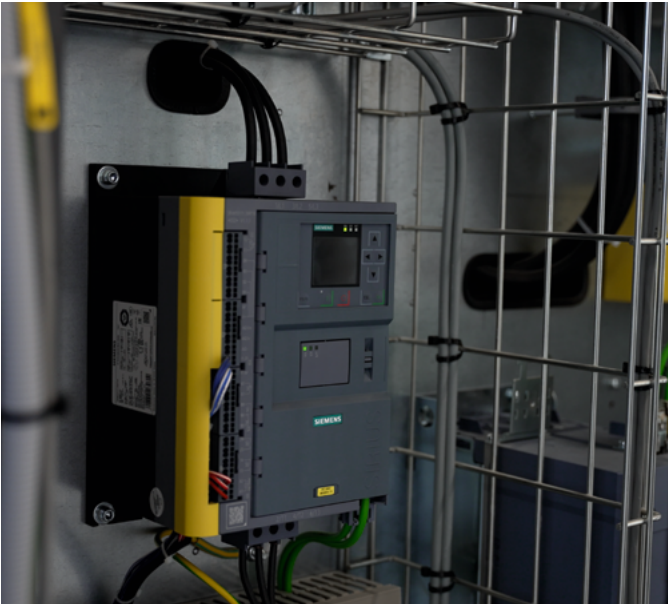
To reduce the strain on machine parts in the Grain Innovation Center, compact Sirius 3RW soft starters allow the electric motors to start up gently.
