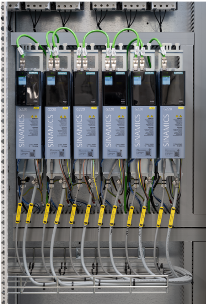
Sinamics G220 frequency inverters master heavy starting and optimize process parameters – even for small test samples in the Grain Innovation Center.
