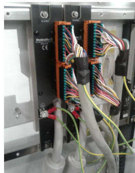
Downtime was minimized by plugging the APACS+ MTA cables into the FAD Adapters.
