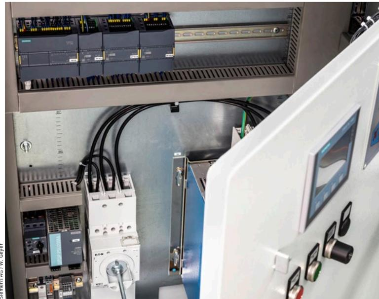
Simatic S7-1200 in the CPU1214 FC version can be extended by up to eight standard or fail-safe signal modules – and exactly meets Dalex's requirements and needs
