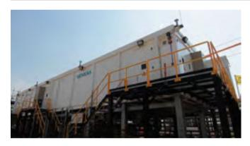
Siemens has supplied customized, fully equipped, and pre-tested modular E-Houses to a Colombian company that transports light crude oil, intermediate blends, and heavy crudes. The E-Houses, which ensure the fast, reliable power supply on oil rigs, include the comprehensive portfolio of medium- and low-voltage switchgear as well as busbar trunking systems.
