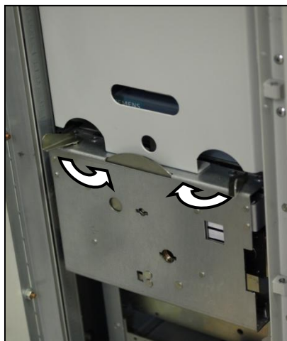
Fig. 233: Interlocking the contactor truck
