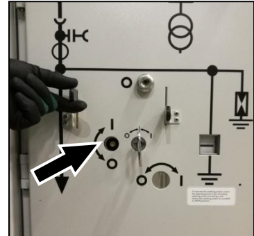
Fig. 180: Operating shaft for racking crank
