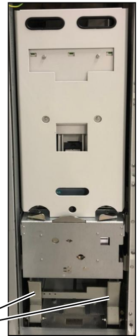
Fig. 225: Contactor panel with high-voltage door open
