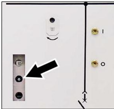
Fig. 43: Position indicator of circuit-breaker on high-voltage door
