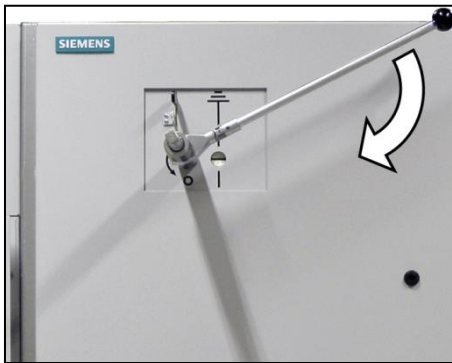
Fig. 345: Closing the busbar earthing switch
