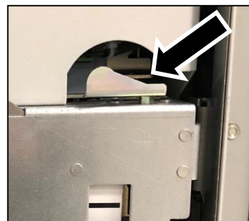
Fig. 234: Contactor truck locked
