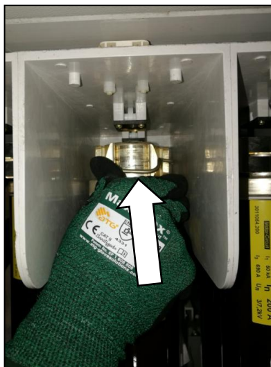
Fig. 246: Opening the fuse-link bracket in the striker area (operating side of contactor truck)
