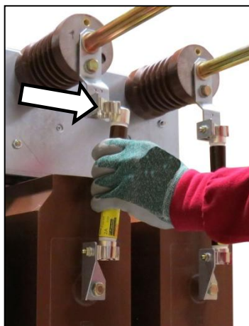
Fig. 257: Pulling off the upper end
