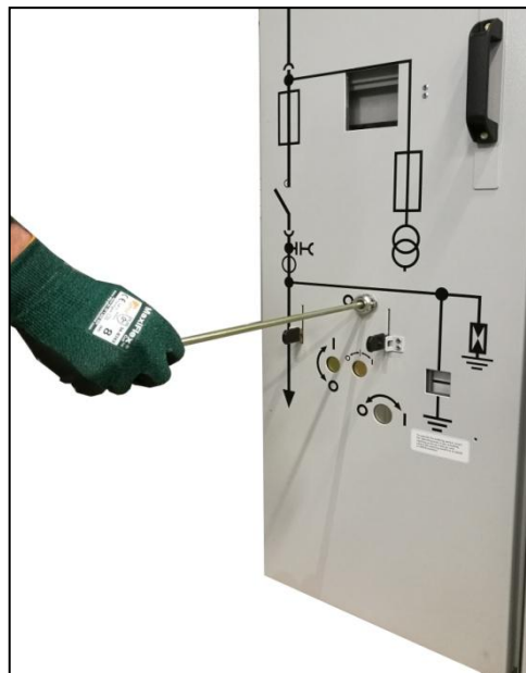
Fig. 186: Push rod inserted
