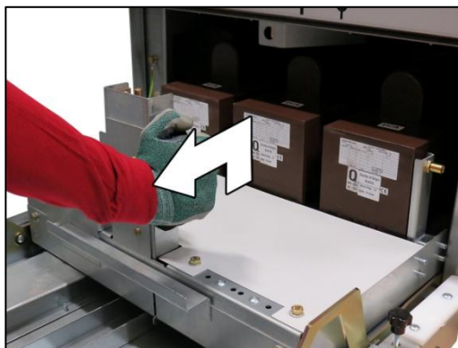
Fig. 294: Pulling the voltage transformers onto the service truck
