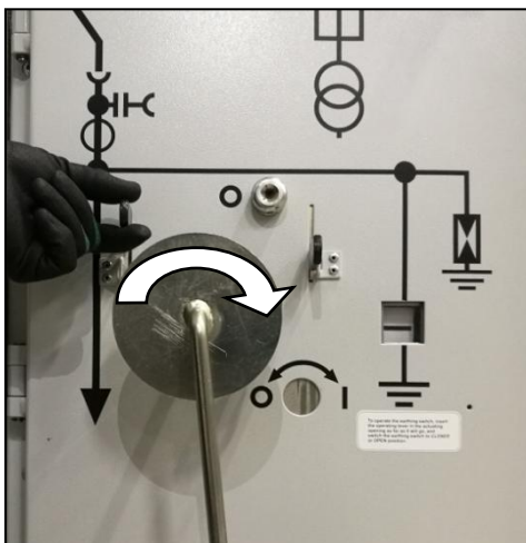
Fig. 174: Turning the racking crank clockwise
