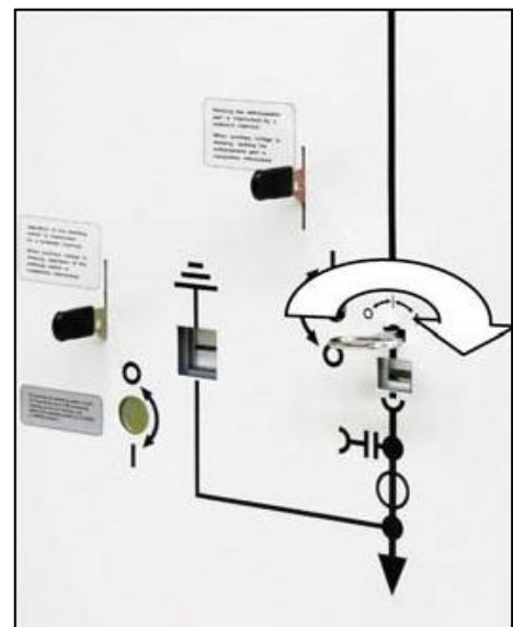
Fig. 48: Turning the double-bit key clockwise
