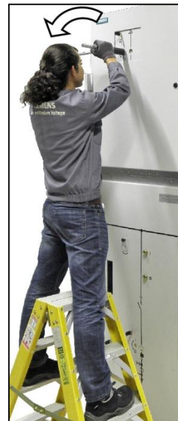
Fig. 359: Opening the busbar earthing switch using an electrician's ladder
