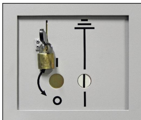
Fig. 352: Operating slide on busbar earthing switch padlocked
