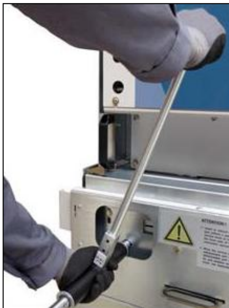
Fig. 120: Operating the feeder earthing switch operating shaft
