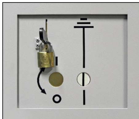
Fig. 349: Operating slide on busbar earthing switch padlocked
