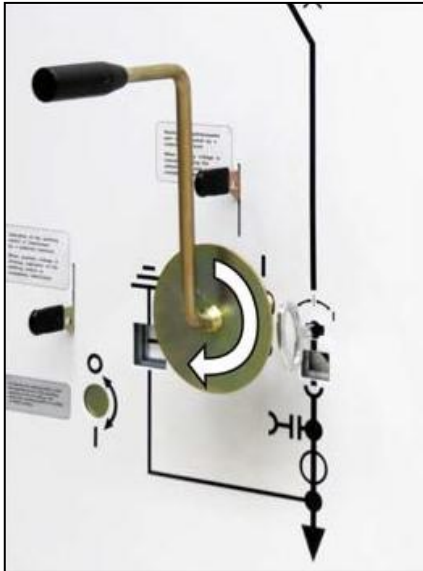
Fig. 49: Turning the racking crank clockwise
