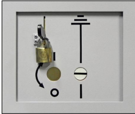
Fig. 362: Operating slide on busbar earthing switch padlocked
