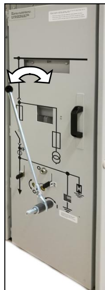
Fig. 212: Turning the lever to the right and left alternately
