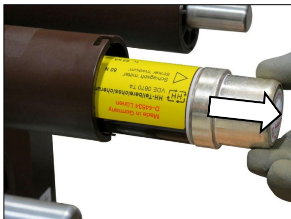
Fig. 320: Pulling the fuse-link out
