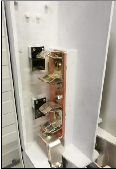
Fig. 240: HV HRC fuse-link removed in the striker area
