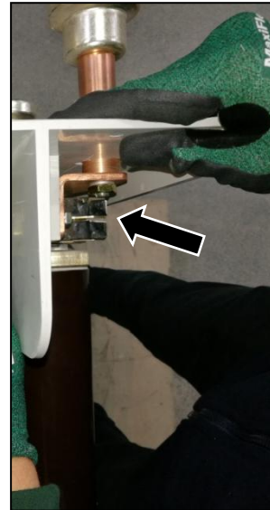
Fig. 241: HV HRC fuse-link removed on the opposite side of the striker area
