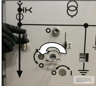
Fig. 179: Turning the double-bit key counter-clockwise
