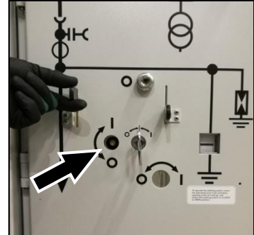
Fig. 173: Operating shaft for racking crank
