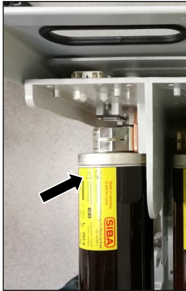
Fig. 244: HV HRC fuse-link inserted and fuse-link bracket closed in the striker area
