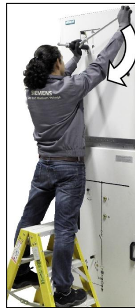
Fig. 346: Closing the busbar earthing switch using an electrician's ladder
