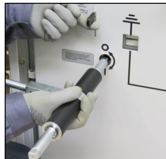
Fig. 89: Inserting lever with pins and openings parallel
