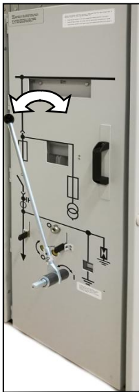
Fig. 204: Turning the lever to the right and left alternately
