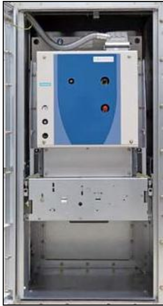
Fig. 105: Circuit-breaker panel with high-voltage door open
