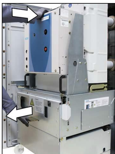
Fig. 126: Pushing the withdrawable circuit-breaker into the panel
