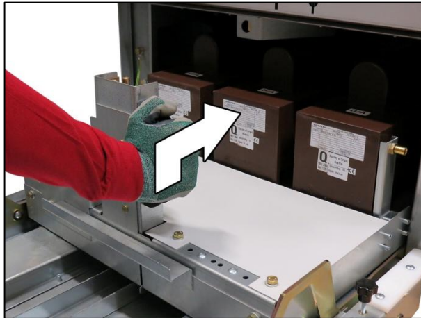
Fig. 302: Pushing the removable voltage transformers into the panel
