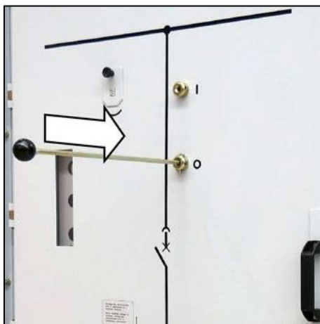
Fig. 73: High-voltage door with push rod in the actuating opening
