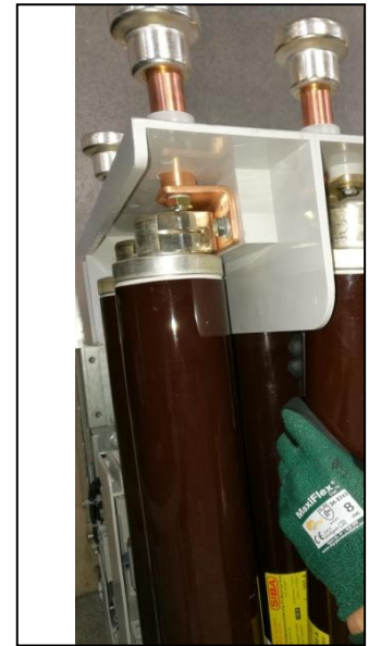
Fig. 245: HV HRC fuse-link inserted and fuse-link bracket closed on the opposite side of striker area
