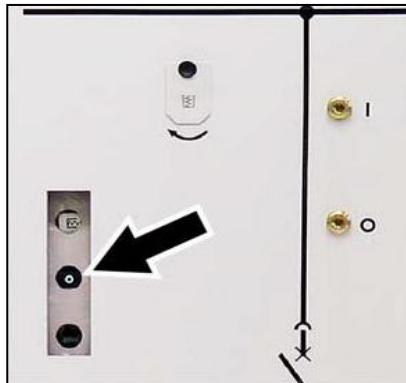
Fig. 52: Position indicator of circuit-breaker on high-voltage door
