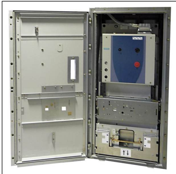
Fig. 133: Circuit breaker panel with high-voltage door open
