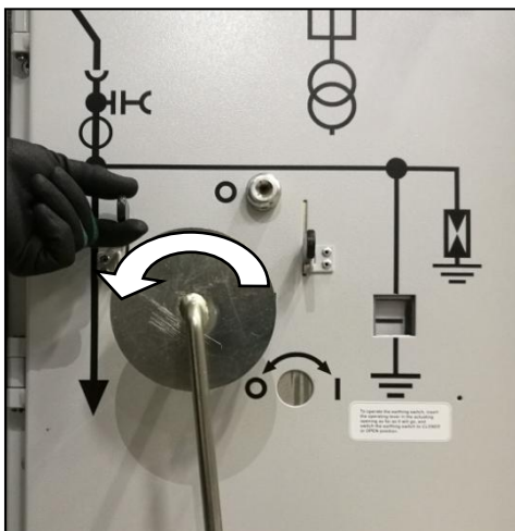
Fig. 181: Turning the racking crank counter-clockwise
