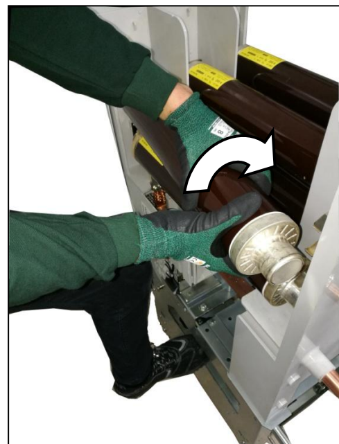
Fig. 243: Inserting the HV HRC fuse-link on the opposite side of the striker area
