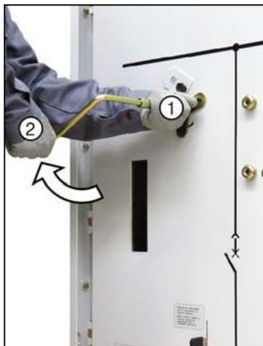
Fig. 82: Hand crank on high-voltage door
