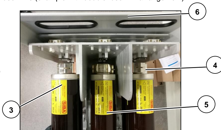
Fig. 236: Seen from top: Arrangement of HV HRC fuse-links (example with double fuse-link arrangement)
