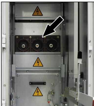
Fig. 387: Shutter to the connection compartment open
