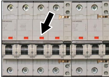
Fig. 157: Miniature circuit-breakers switched on, indicators red
