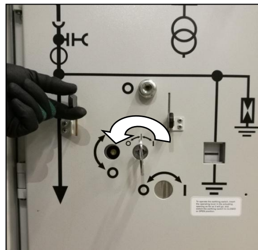
Fig. 182: Turning the double-bit key counter-clockwise
