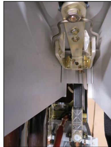
Fig. 249: HV HRC fuse-link removed on the opposite side of the striker area
