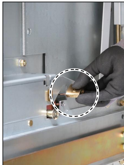
Fig. 369: Padlocking the shutter mechanism on the left side in the switching-device compartment
