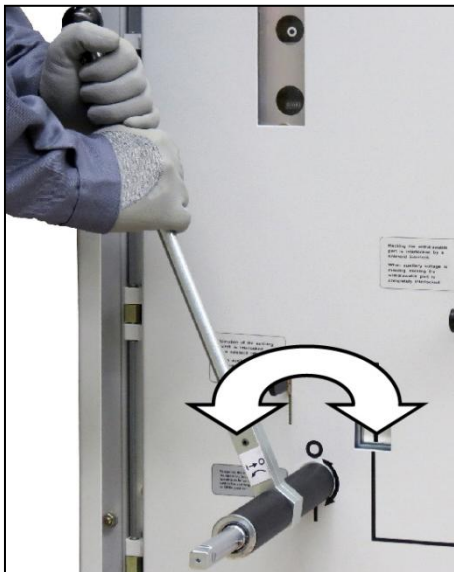
Fig. 98: Turning the lever to the right and left alternately Fig. 99: Position indicator on high-voltage door in OPEN position
