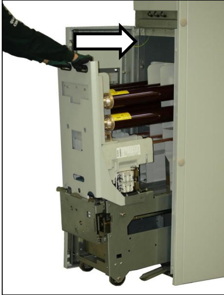
Fig. 231: Pushing the contactor truck at the top into the panel
