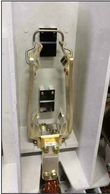
Fig. 248: HV HRC fuse-link removed in the striker area
