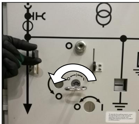
Fig. 194: Turning the double-bit key counter-clockwise
