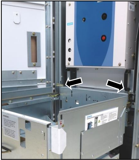
Fig. 110: Unlocking the withdrawable circuit-breaker
