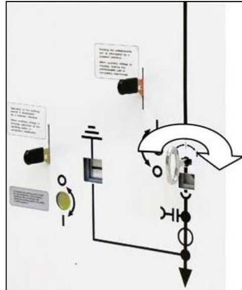
Fig. 50: Turning the double-bit key clockwise
