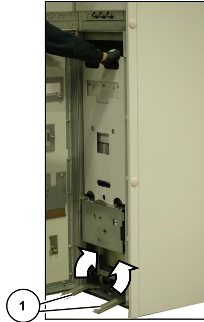
Fig. 232: Lifting the ramps
