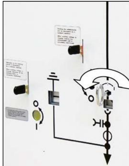
Fig. 59: Turning the double-bit key counter-clockwise
