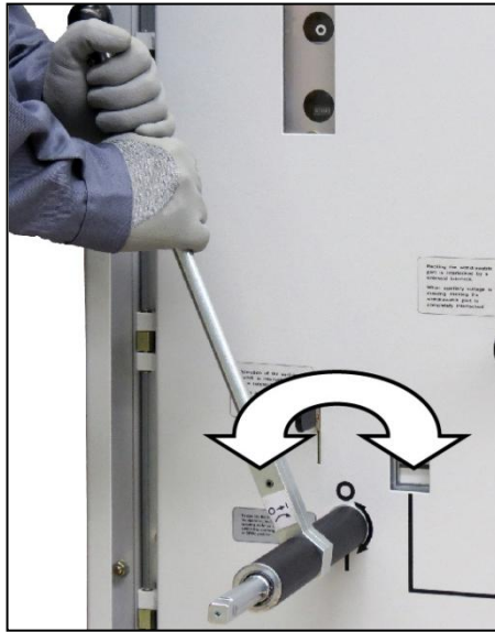
Fig. 90: Turning the lever to the right and left alternately
