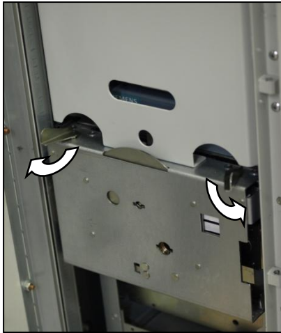
Fig. 218: Releasing the interlocking with the panel
