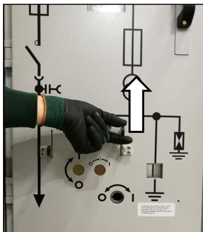
Fig. 208: Lifting the operating slide
