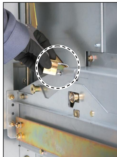
Fig. 364: Padlocking the shutter mechanism on the right side in the switching-device compartment
