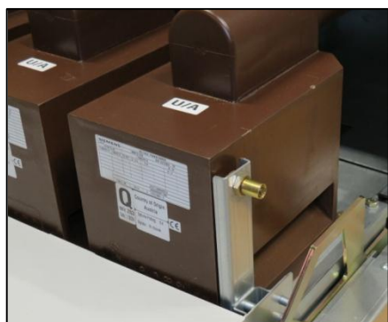
Fig. 308: Rating plate on removable voltage transformer
