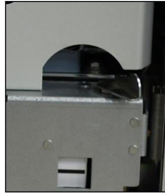
Fig. 219: Contactor truck unlocked
