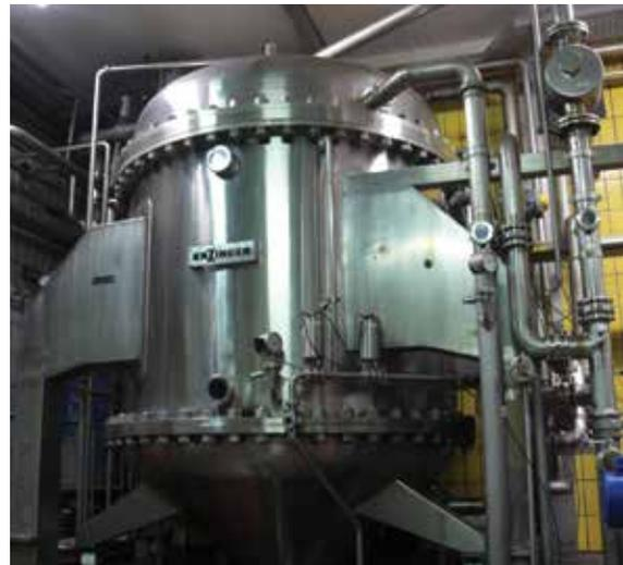
Filter cellar with clamp-on flow meter, hose pump (blue) and Kieselguhr tank (open)
