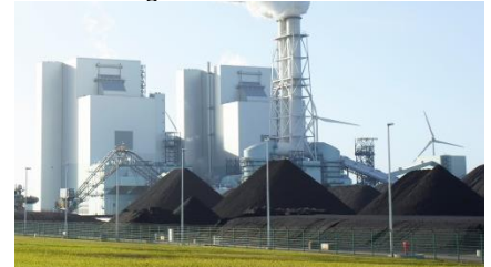
Eemshaven steam power plant.
