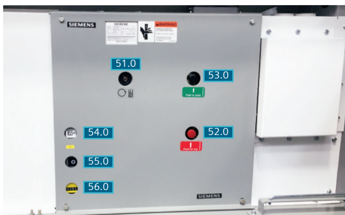
Figure 9: Operator panel controls of the circuit breaker and manual charging of closing spring
