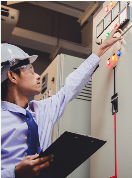
Engineer checks voltage in control panel.
