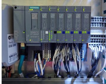
Another was a dairy application needing it to run a series of valves, pumps, and flow meters – 30 I/O points in all and a combination of digital and analog throughputs.
