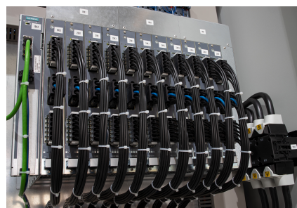
A compact and high-performance solution: Vesper can integrate a great deal of functionality in a small space thanks to a SIMATIC ET200SP controller (top) and an HCS heating control system
