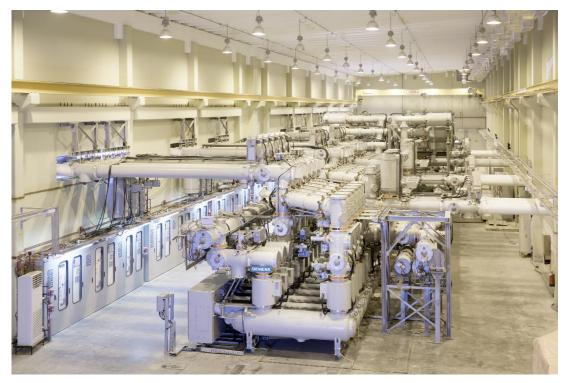
Comparable 380 kV 8DQI gas-insulated switchgear will boost the transmission capacity of the Daxlanden substation and are an important part of covering the increased transport demand in German high voltage grid.
