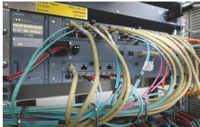
Image 1: Redundant 10-gigabit backbone for an efficient, soon-to-be virtual process control: One of two rack-mountable Industrial Ethernet switches/routers SCALANCE XR552-12M from Siemens.
