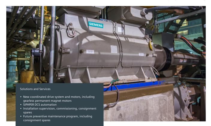
the space on the drive side of the machine prohibited a traditional approach. To answer the challenge, Siemens provided gearless permanent magnet motors that allowed the needed space for operations and maintenance. The ability to reduce the footprint by eliminating gearboxes proved an important feature in a retrofit where every foot counted. In addition, the Siemens Customer Service group provided services and spares for the repurposed old equipment.
