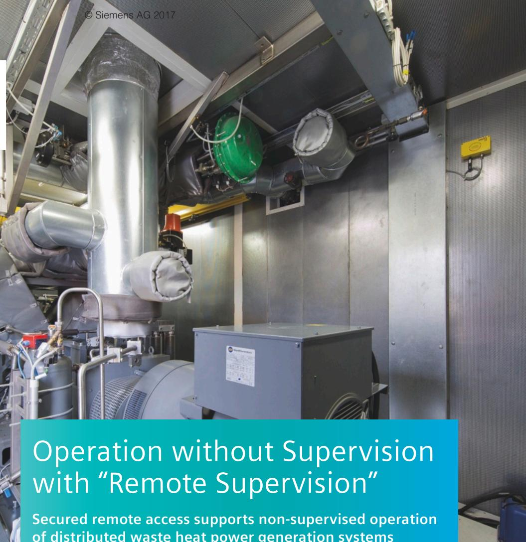
Contrary to the standard solution with flue-gas evaporators, the waste heat is transferred through a thermal oil system to the ORC fluid bioethanol. The fluid is compressed by means of a feed pump and conveyed in a loop. The energy from the waste heat source is transferred in a heat exchanger to the fluid, whereby vaporizes and overheats it.
