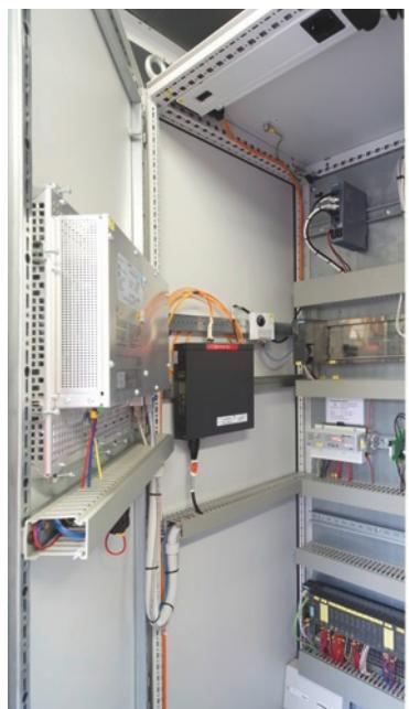
A SCALANCE S615 security module (above) is the link between the plant and SINEMA Remote Connect; this module is easily integrated into existing networks and protects the lower-level parts of the system against unauthorized access.
