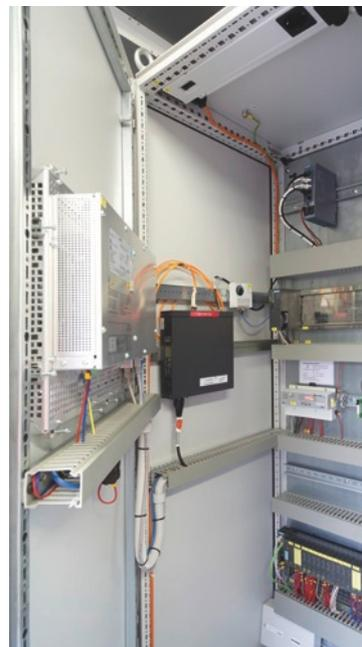
A SCALANCE S615 security module (above) is the link between the plant and SINEMA Remote Connect; this module is easily integrated into existing networks and protects the lower-level parts of the system against unauthorized access.
