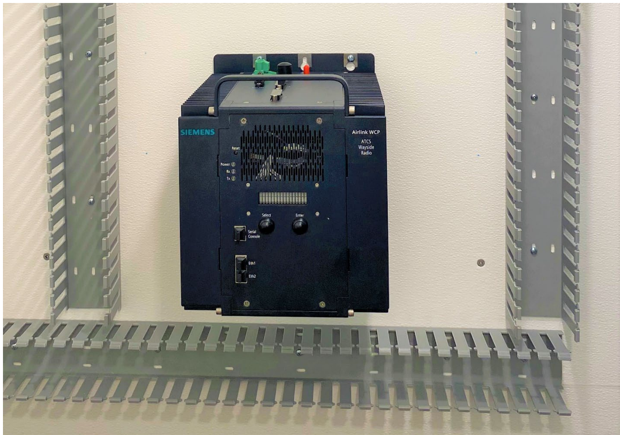
Figure 4-6 Typical Airlink WCP Wall Installation – Front View
