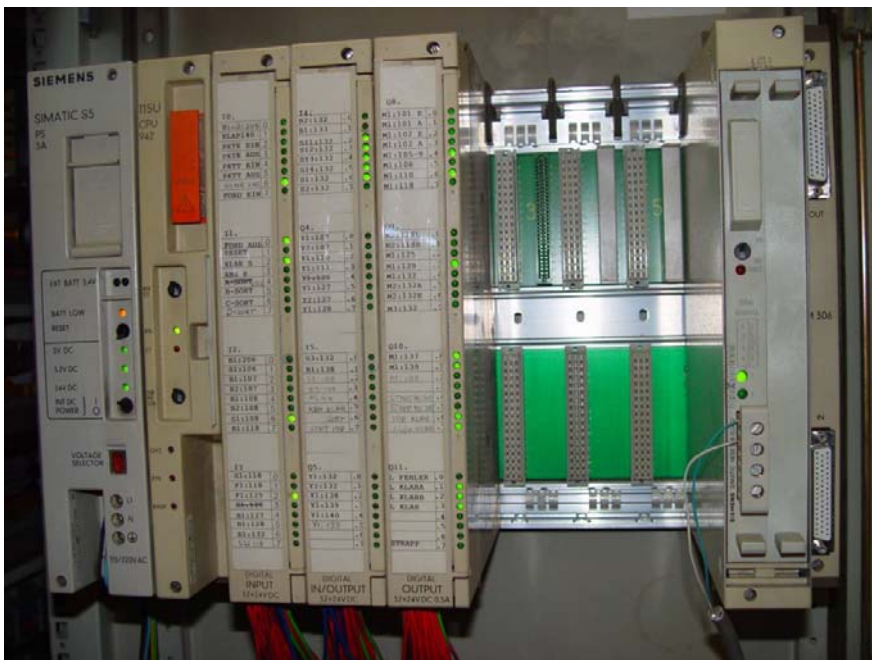
Figure 1-5: Control unit of the «MIGHOLZ» wood-processing machine
