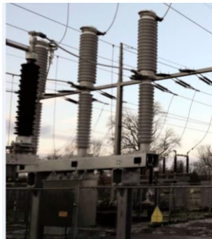
145 kV Blue Circuit Breakers, LT 30 in operation in GER, POL since 2018 15 ordered in NOR, SWE, GER, SUI, GBR, POL, ROM, KAZ, USA
