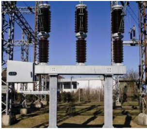
72,5 kV Blue Circuit Breakers, LT 6 in operation in FRA, LUX, DEN, AUS since 2010
