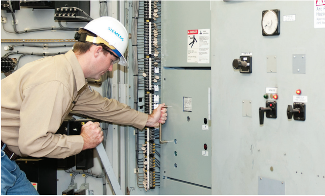
Before: Original floor-mounted lever racking, commonly used on types D and F switchgear, required the operator to stand in front of the breaker with the panel door open.
