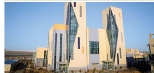
Ansan, South Korea SCC6-8000H 2x1 combined cycle plant
