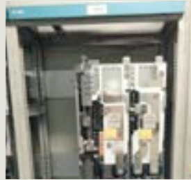
3. Install chassis, connect to DC busbar
