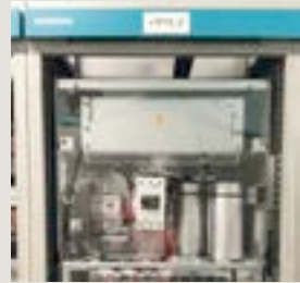
2. Install SINAMICS filter – AIM
