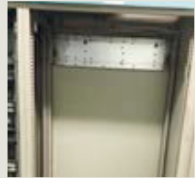
4. Re-align the DC busbar position
