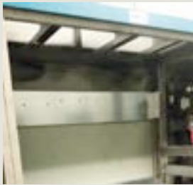
1. Install SINAMICS chassis supporting mechanics
