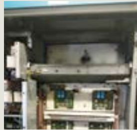
3. Remove chassis and supporting mechanics
