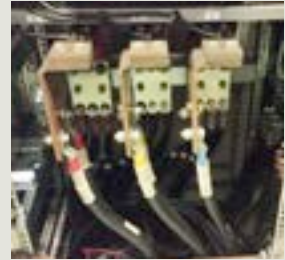
4. Connect motor cables and communication wiring
