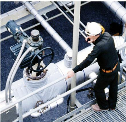
providing input to the valve position was “drifting” with changes in temperature and vibration. Recalibration did not solve the control problem.
