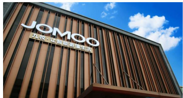
Exterior of JOMOO five-star customization experience shop
