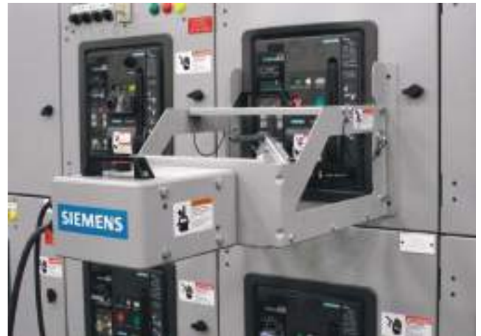
Remote Racking Device
