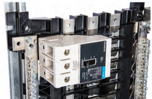
Example of Back-fed NGB Main breaker installed
