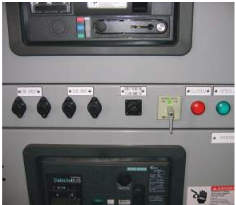
Control port on WL Switchgear
