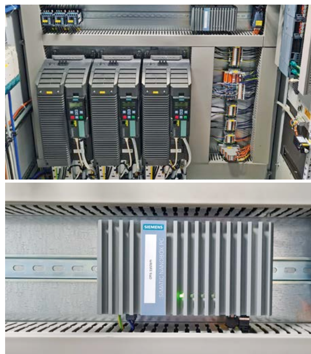
Figure 2: Cabinet with SINAMICS G120C drives and Industrial Edge PC (SIMATIC IPC227 NANOBOX PC)
