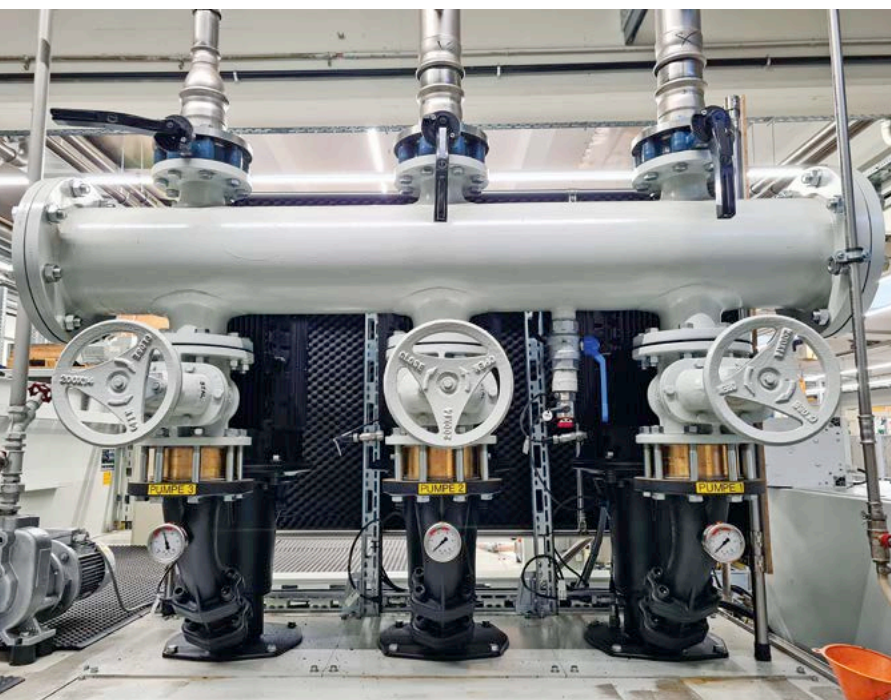
Figure 1: Filter and pump application for cooling lubricant in Bad Neustadt factory
