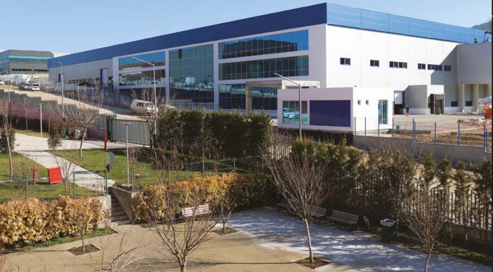
Schott has invested roughly €9 million in its expanded plate glass facilities, including state-of-the-art production technology and a digital infrastructure. Image source: Schott AG.
