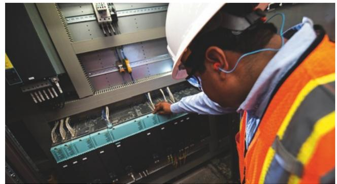
In the plant's upgraded and expanded network more than 4,000 production-related devices, plus 1,500 Siemens SINAMIC G120 drives are connected.
