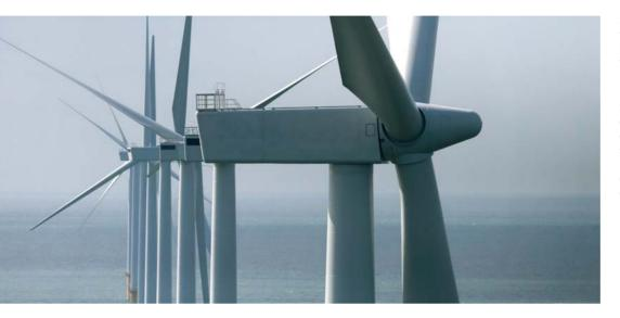
25 wind turbines from Siemens are in operation in the Burbo Offshore Wind park off the coast of Liverpool. The wind power plants, of type SWT-3.6-107, have an output of 3.6 megawatts each. The wind park supplies 80,000 households with eco-friendly electricity and has a total capacity of 90 megawatts.
