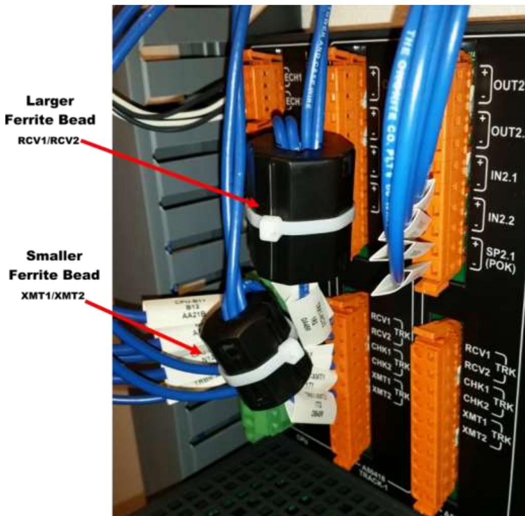
Figure B-14 Ferrite Bead Sizes
