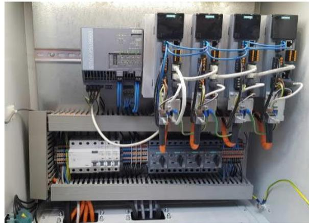
Equip the material feeding conveyor for the new SINAMICS S120 Motor Module production line in MC Factory Erlangen F80. The S210/ S-1FK2 drive a linear axes. The linear axe lifts and positioned the roller conveyor **1** which is attached to it. In total there are 4 conveyor stations with each 4 lifters. Products used: SINAMICS S210 Servo Drive System and SIMATIC ET200 SP open controller. Please see application video [here](#)
