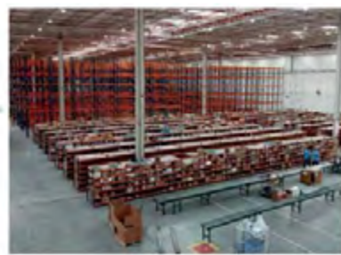
JundTech distribution center (Jundiaí, SP)
