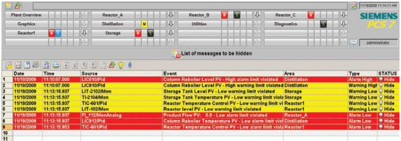
Figure 9 – HMI list of shelved alarms
