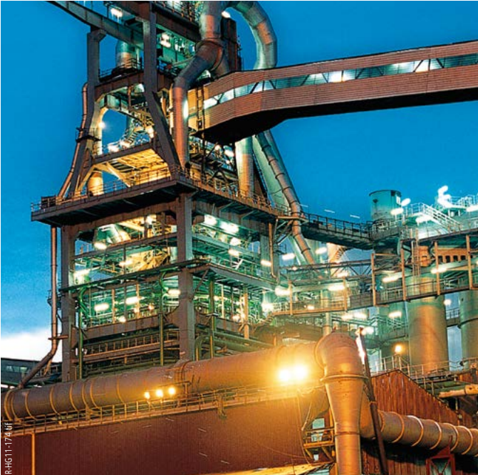
Industrial application: Refinery
