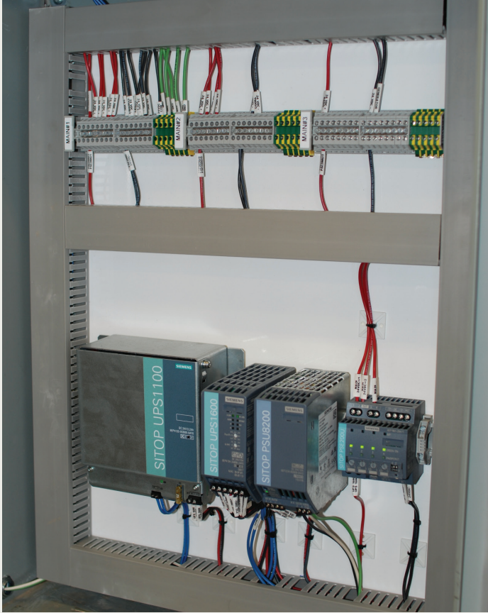
The SITOP UPS1600 24 V DC UPS at EPWater installed with UPS1100 battery, SITOP PSU8200 power supply and PSE200U for additional circuit protection
