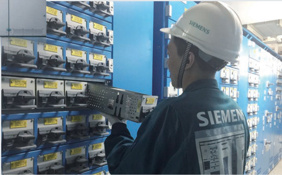
SIVACON 8PT低压配电柜 SIVACON 8PT Low Voltage Switchboard
