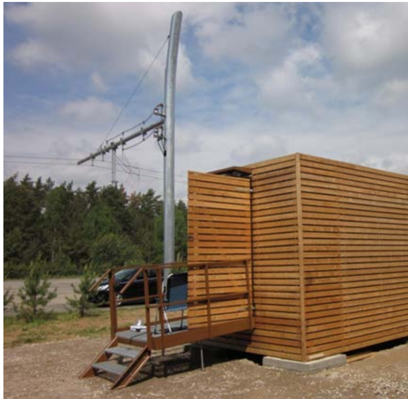
Highway substation in prefabricated steel-enclosed container – exterior wood facing
