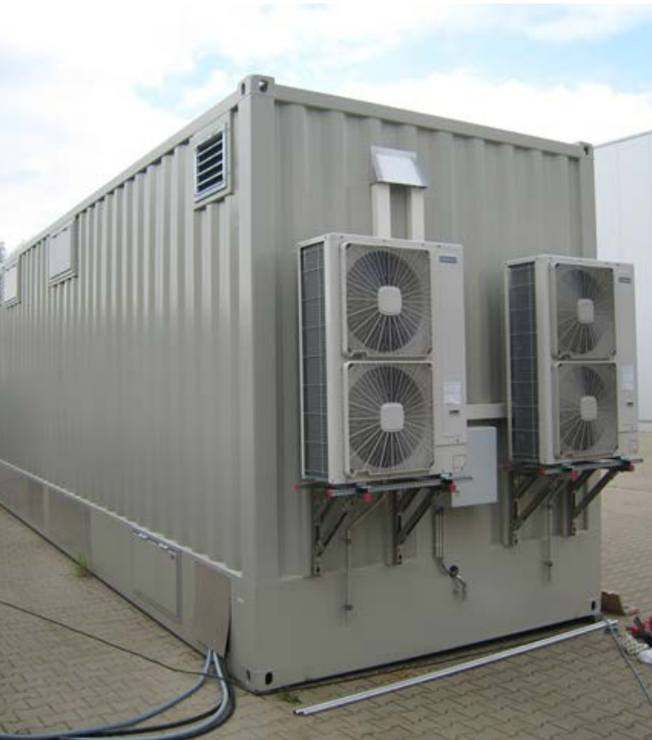
Substation prefabricated in the form of a steel-enclosed container
