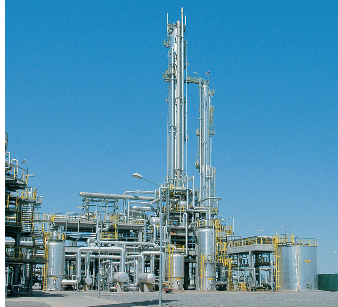
A state-run fertilizer manufacturer in Tedjen, Turkmenistan decided in favor of an automation system from Siemens. The order also included engineering, installation and system testing.
