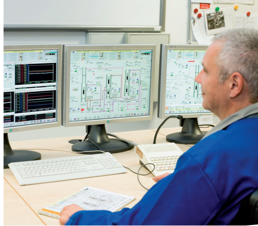
At BASF in Ludwigshafen, Germany, material flow is controlled through valves, in some cases with positioners. Overall monitoring of the ammonia plant takes place in the central control room.
