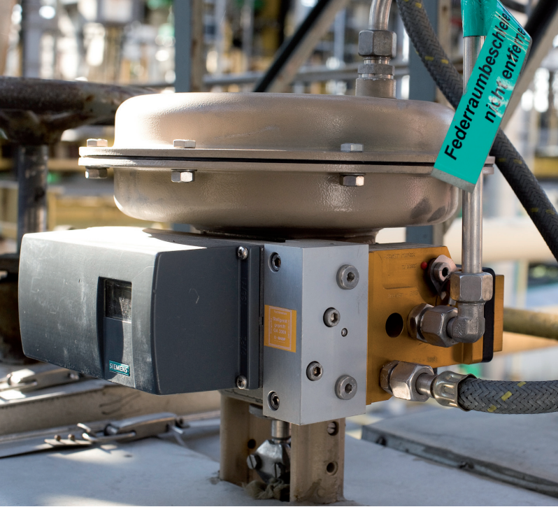
At BASF in Ludwigshafen, Germany, material flow is controlled through valves, in some cases with positioners. Overall monitoring of the ammonia plant takes place in the central control room.
