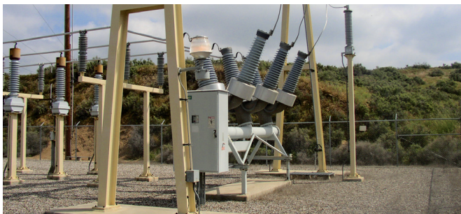
Siemens TCP145 kV 40 kA SF 6 circuit breaker
