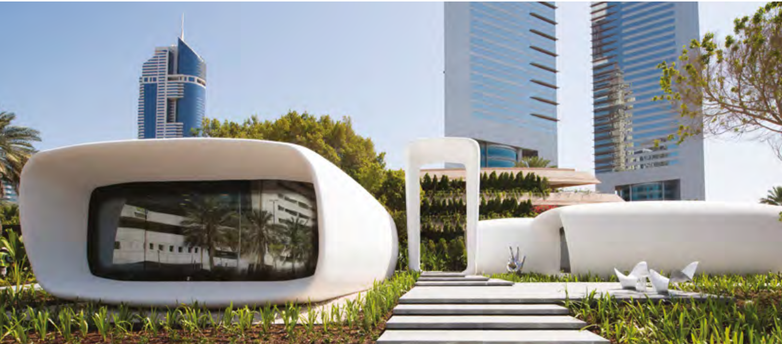
Copyright: Dubai Future Foundation. The world's first office building produced by a 3D printer opened in Dubai. The 250-square-meter “Office of the Future” was built using a 3D printer measuring 20 feet high, 120 feet long and 40 feet wide, and erected near the Emirates Towers in Dubai. The building technology with access control and surveillance systems was provided by Siemens and is integrated into a central building management platform. The technology ensures low operating costs and reduced energy consumption.
