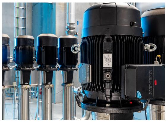
When fitted with Simotics Connect 400, size AH100 to AH450 low-voltage motors can be analyzed using the cloud-based Sidrive IQ Fleet App.
