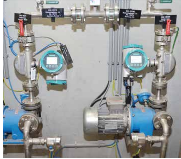
The SITRANS FC430 measuring the correct dosage of the additives as well as the denatured alcohol.
