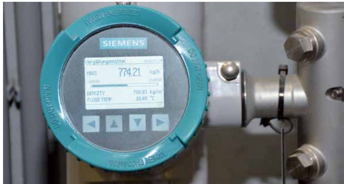
The new Siemens SITRANS FC430 Coriolis flow meter in use at the Donau Chemie Group.
