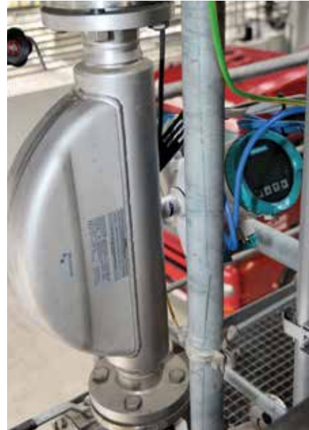
The SITRANS FC430 measuring the correct dosage of the additives as well as the denatured alcohol.
