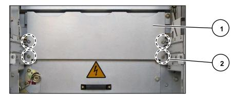
Fig. 158: 4 bolted joints on protection plate of switching-device compartment.
