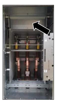
Fig. 103: Busbar cover installed
