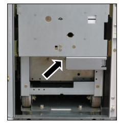
Fig. 298: Front view of withdrawable circuit-breaker
