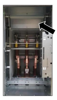
Fig. 56: Panel prepared for accessing the busbar compartment
