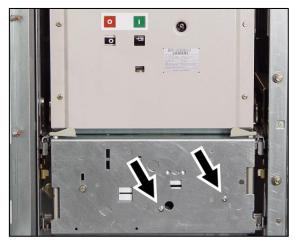
Remove 1 locking bolt of the solenoid interlock at the switching-device truck of the contactor panel with panel width 435 mm
