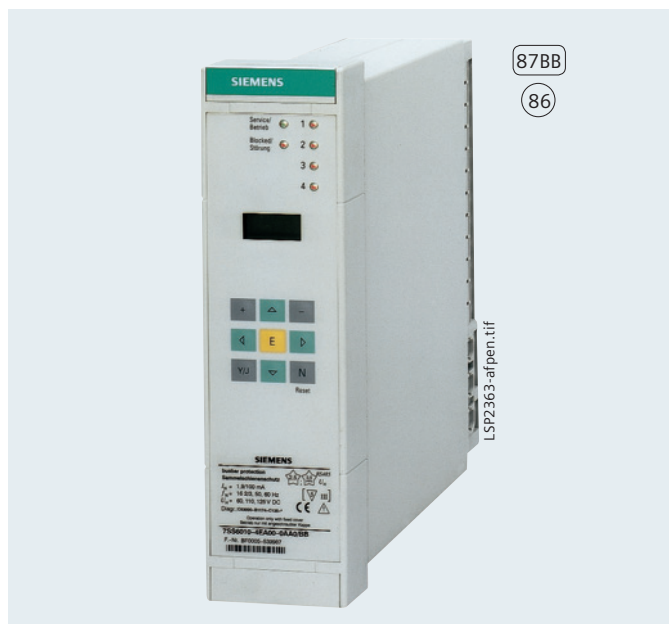
Fig. 9/1 7SS601 measuring system
