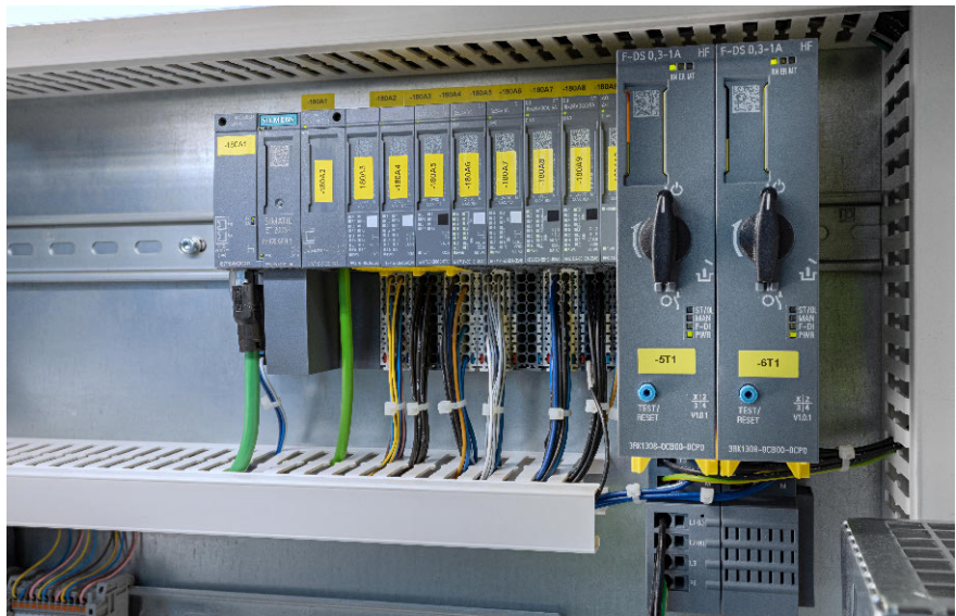
Figure 1 The compact, fail-safe ET 200SP motor starters permit more space in the control cabinet due to their small module width of only 30 mm and can be configured quickly and easily in the TIA Portal. Source: Siemens AG
